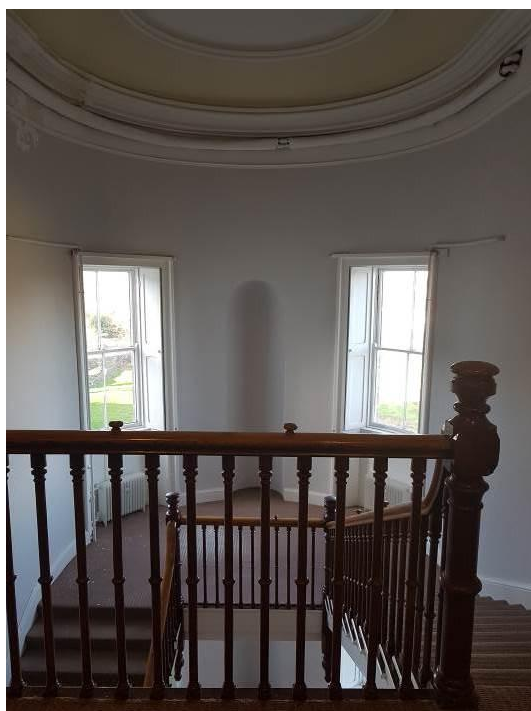
Plate 7.9.1: The existing open-well staircase in the central bay will be safeguarded (2023 image for context)
