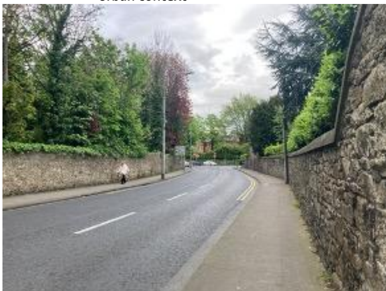
Plate 7.3.12: Milltown Road, due north towards junction with Sandford/ Clonskeagh Roads
