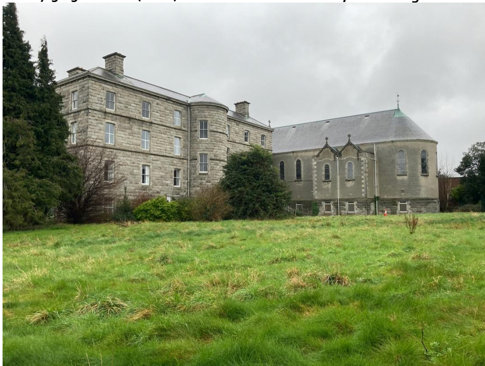
Plate 7.3.26: West (rear) elevation of Tabor House, in context with the Chapel
