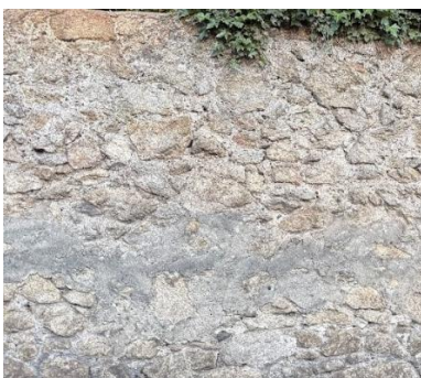
Figure 7.5.5.: Detail of masonry condition to Sandford Road length of wall , which will be repaired and repointed
