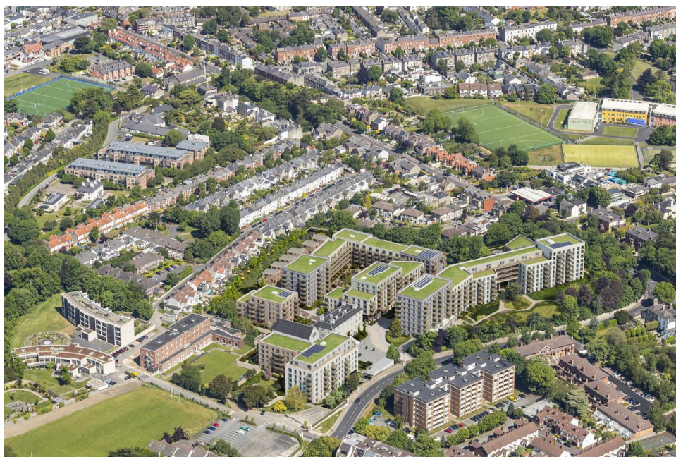
Figure 7.5.1.: Birds eye view of the Chapel and Tabor House in context with the proposed development, as extracted from Aerial Views, 3D Design Bureau
