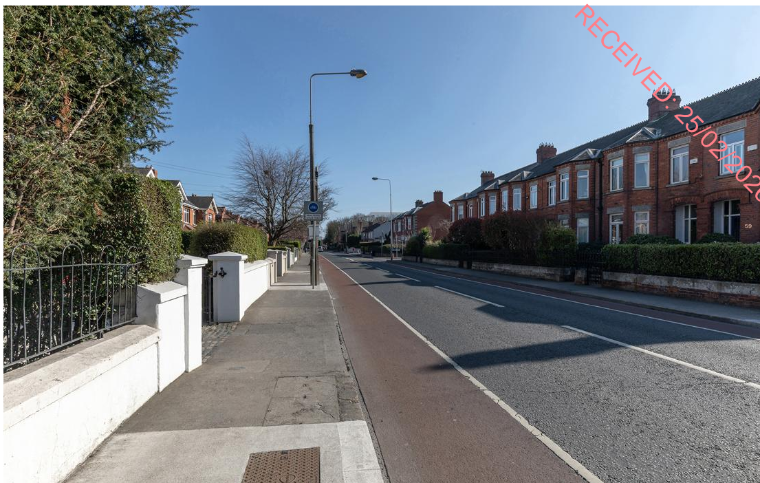
Plate 7.9.5: Verified View, View 1, indicating the marginal visibility of Block A1 above the treeline, from Sandford Road, to the north of the ACA
