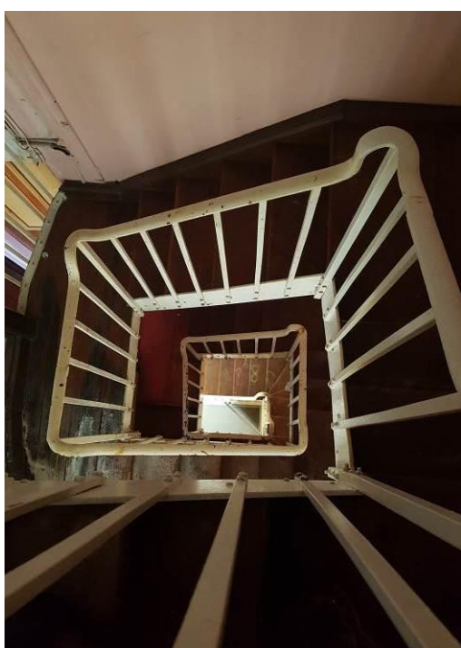
Plate 7.9.3: The secondary stairs in the south of Tabor House will be removed to facilitate the revised spatial configuration
