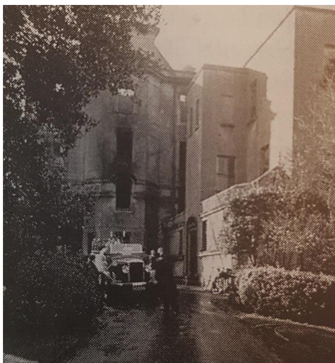
Plate 7.3.22: The fire damaged exterior of the Finlay Wing, indicating its original height of three storey over basement with pitched roof over.
