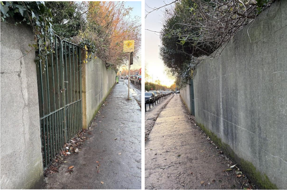
Figure 7.5.6.: Detail of replacement rendered blockwork to Milltown Road length of wall
