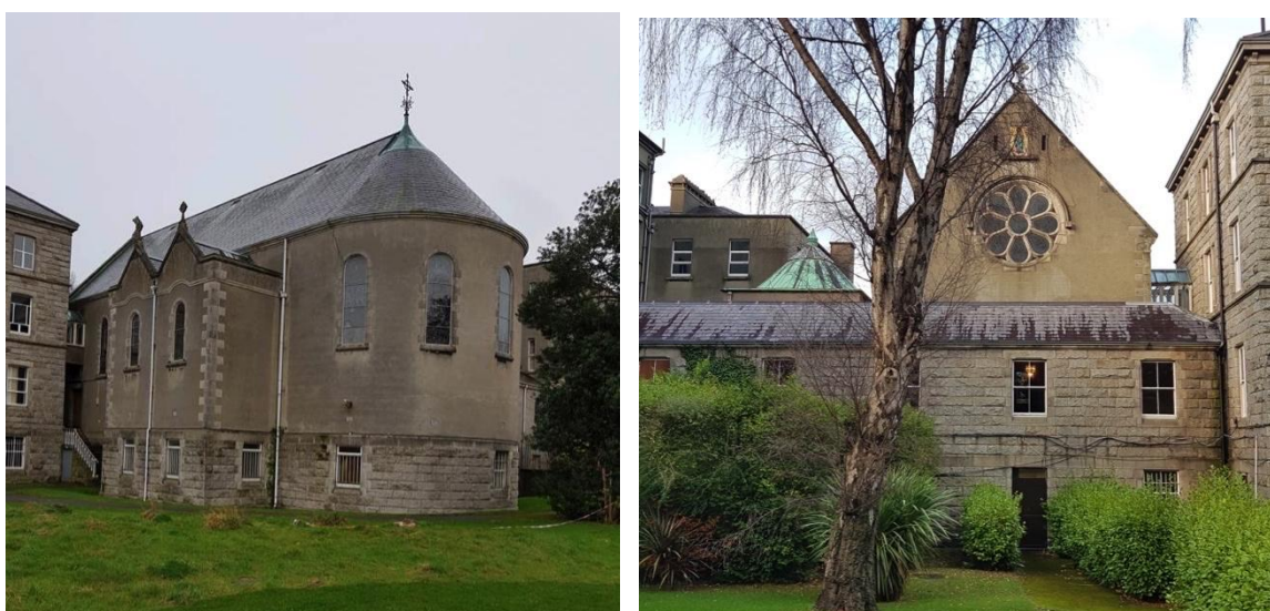
Plates 7.3.27 & 7.3.28: The rear elevation of the Chapel, and the front elevation of the Tabor House Link with gable of Chapel complete with rose window over, image taken in 2023 and included for context
