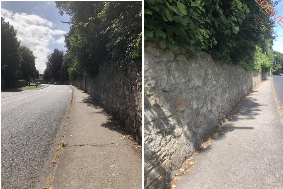
Plate 7.3.30. 31: Boundary wall along Milltown Road
