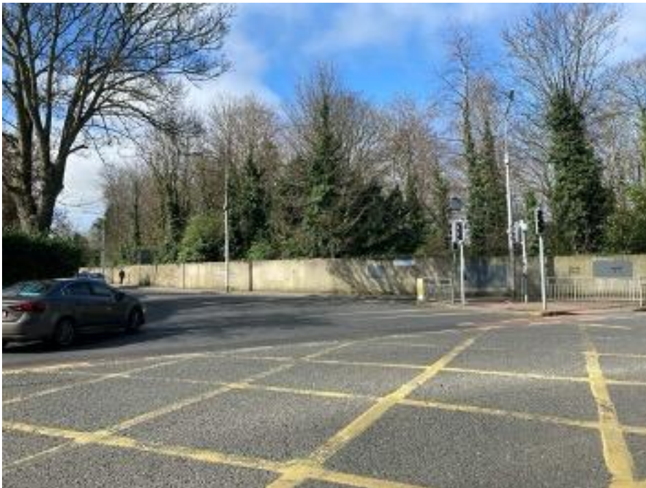
Plate 7.3.32: Replacement section of boundary wall at junction of Milltown and Sandford Roads
