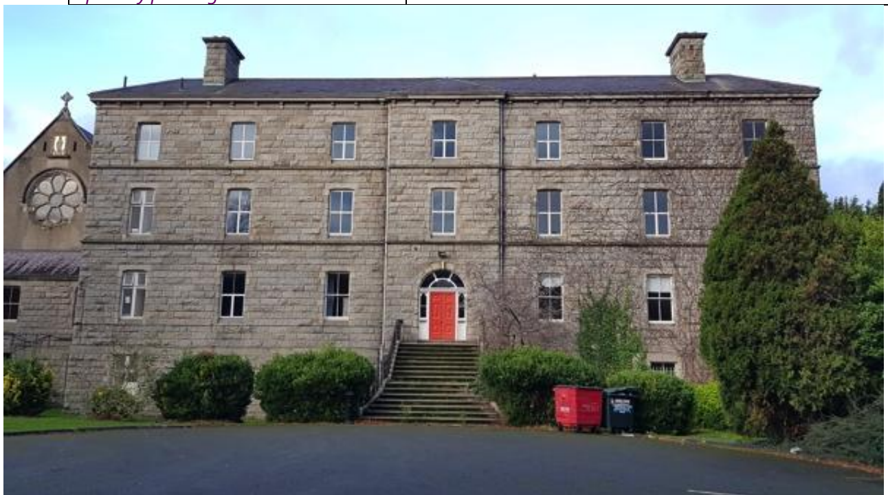
Plate 7.3.25A: East (front) elevation of Tabor House, taken in 2023 and included for context
